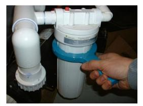
to prevent the water from freezing. Or the water could be drained to avoid damage from freezing. In this case, be sure to loosen both of the couplers that connect the pump assembly to the bowl. This will allow the water in the pipes to be drained that would not be drained by opening the spigot.
