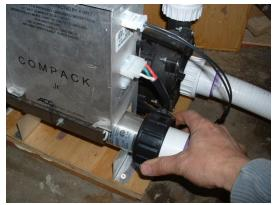
box and clicks into the two retaining arms on the terminal. These arms must be spread apart to remove the connector.
