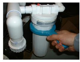
to prevent the water from freezing. Or the water could be drained to avoid damage from freezing. In this case, be sure to loosen both of the couplers that connect the pump assembly to the bowl. This will allow the water in the pipes to be drained that would not be drained by opening the spigot.
